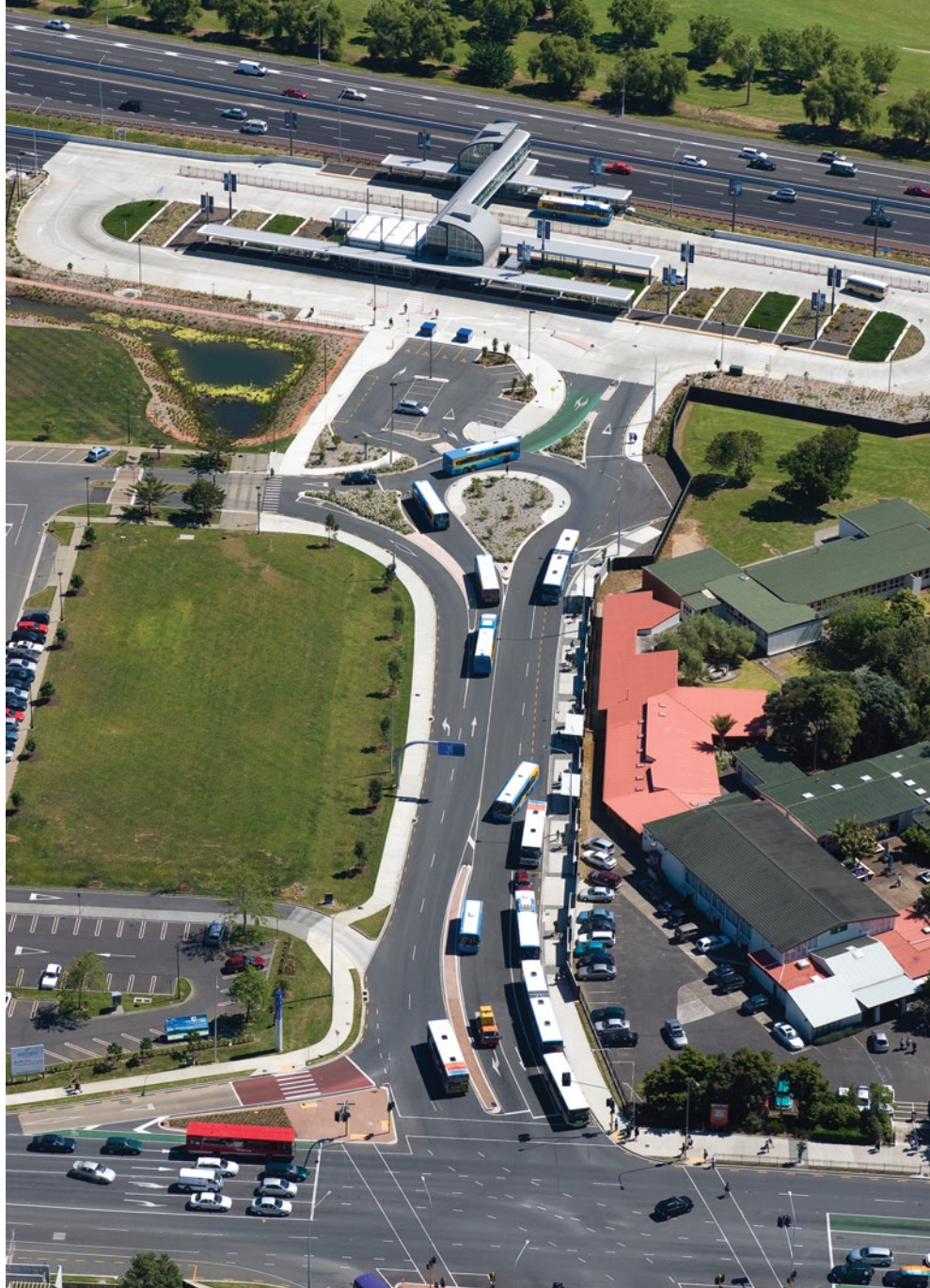
Smales Farm bus station on Auckland's North Shore
