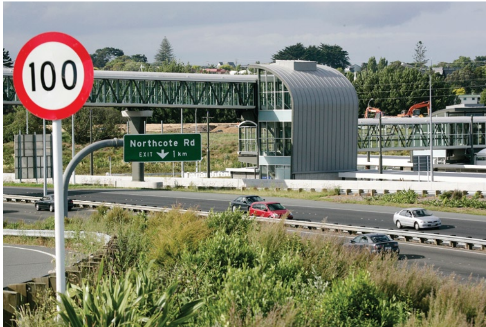
The pedestrian bridge from Akoranga bus station over the Northern motorway (State Highway 1) provides access to AUT's Akoranga campus
