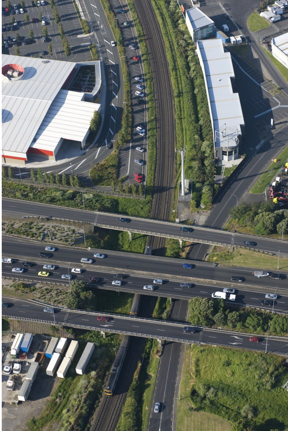
State Highway 1 motorway crossing the Eastern rail line at the Mt Wellington interchange.
