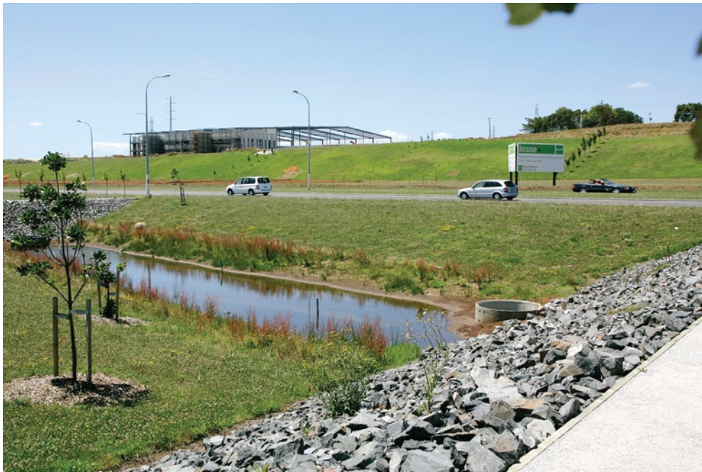
Stormwater swales near Highbrook Business Park, South Auckland illustrate low impact stormwater treatment
