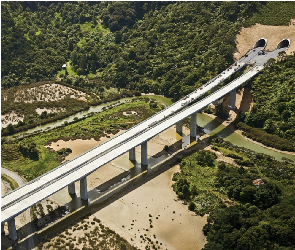
Northern Gateway (a toll route) viaduct crossing the Waiwera River
