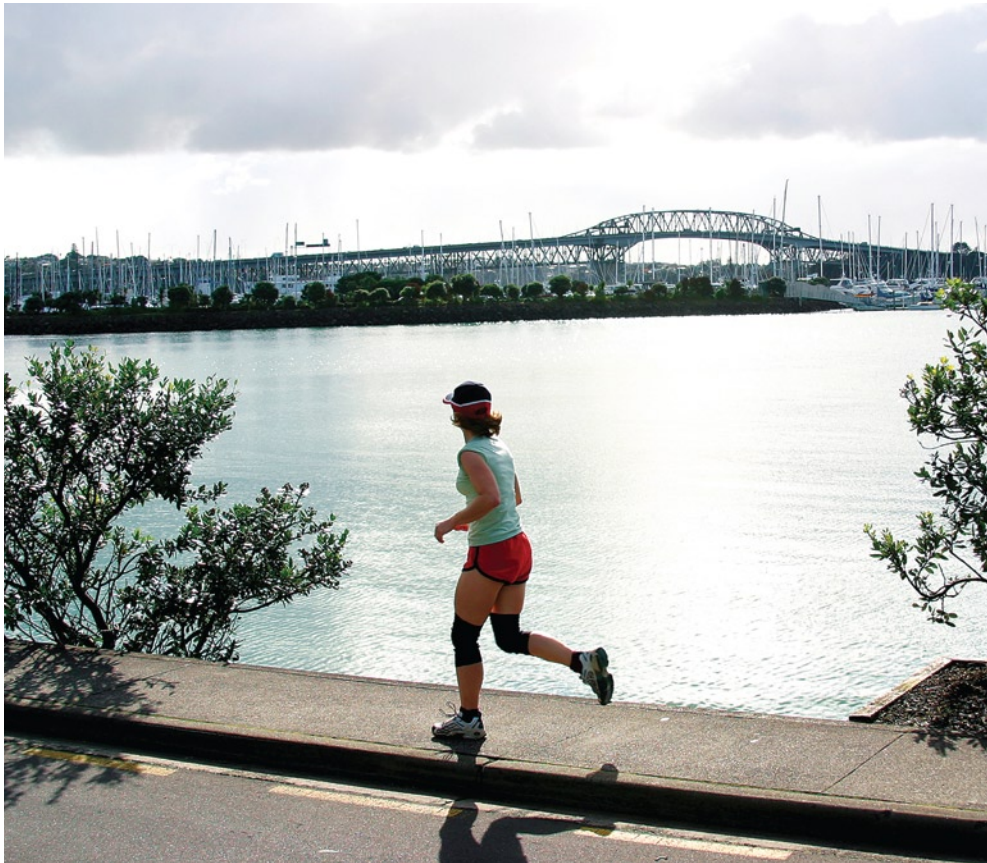
View of Auckland Harbour Bridge (courtesy of Auckland City Council)
