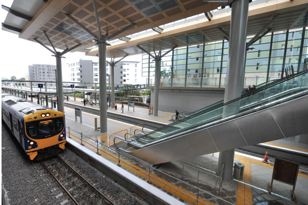
Newmarket rail station
