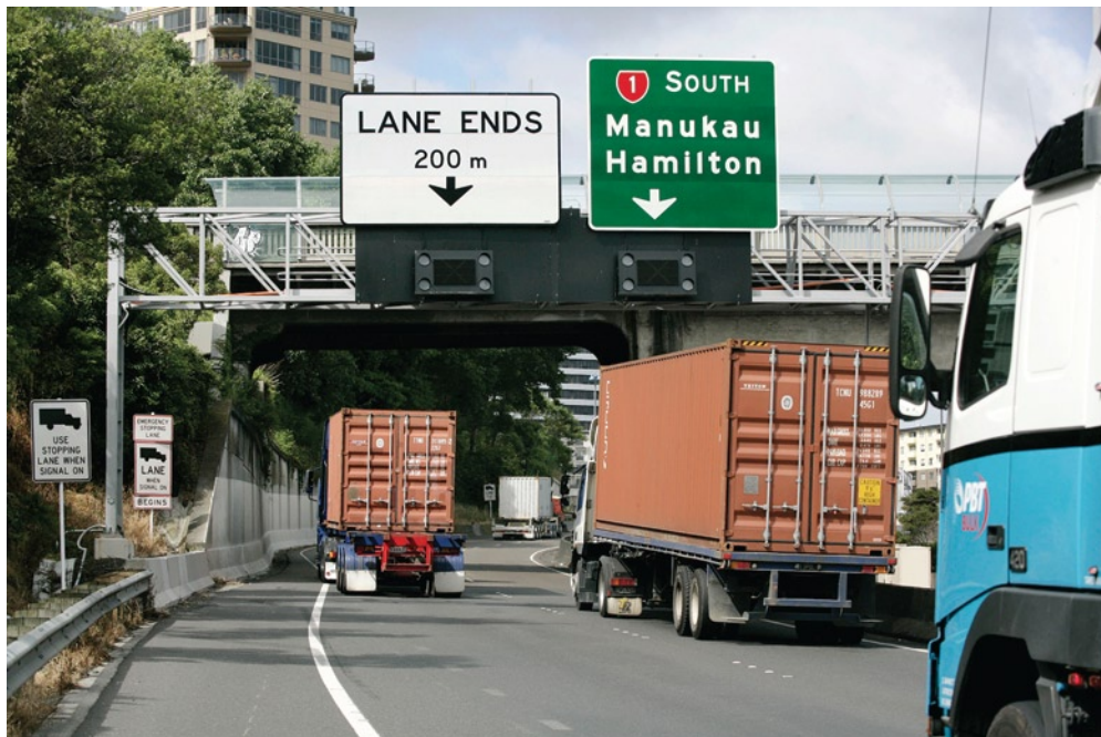
The truck priority lane on Grafton on-ramp eases traffic flow onto the Southern motorway
