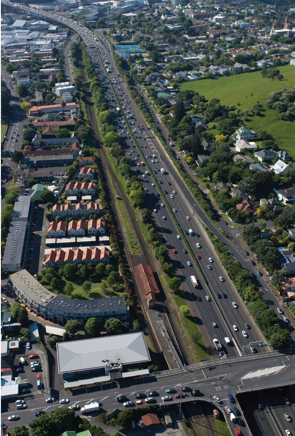
State Highway 1 with Remuera rail station and main trunk line running parallel
